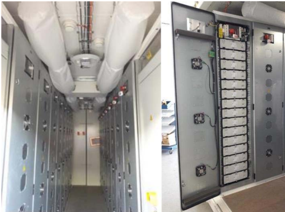
Figure 1 Inside of Intensium Max Container by SAFT
